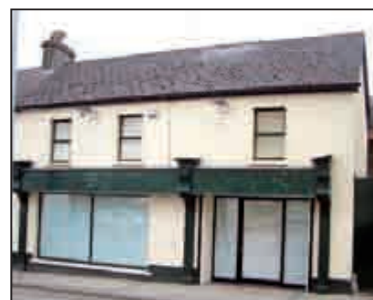
Prime commercial unit to let at Lanesboro Street, Roscommon town.
